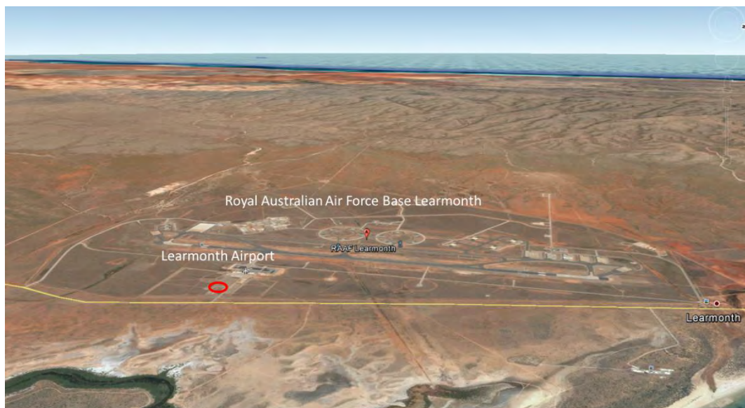
Figure 11. BoM facility at Learmonth airport
