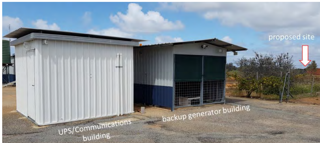
Figure 23. UPS and backup generator adjacent to the proposed site
