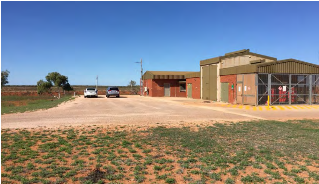
Figure 12. BoM facility at Learmonth airport
