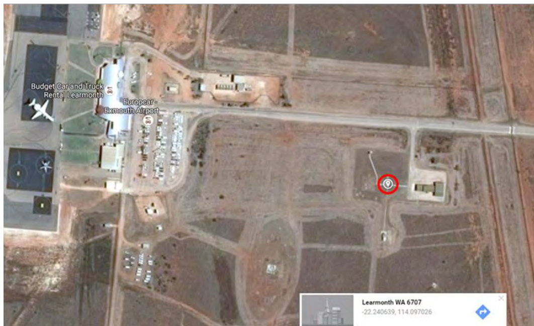
Figure 10. BoM facility at Learmonth airport
