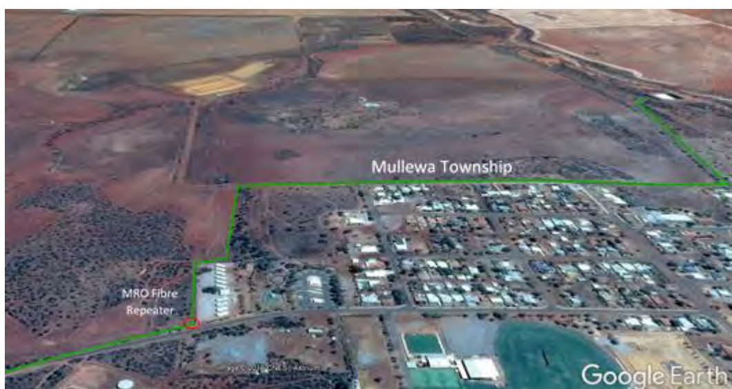
Figure 31. Route of fibre from the MRO and location of fibre repeater hut
